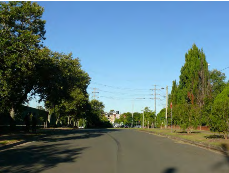
11 Looking to east on Felton Rd
