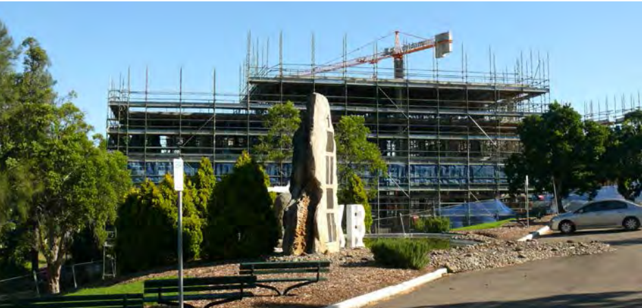
Site photo - under construction
