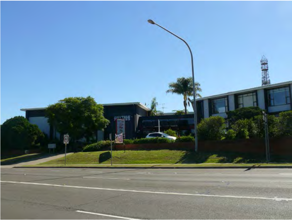
8 Looking to the existing building on site on Pennant Hills Rd
