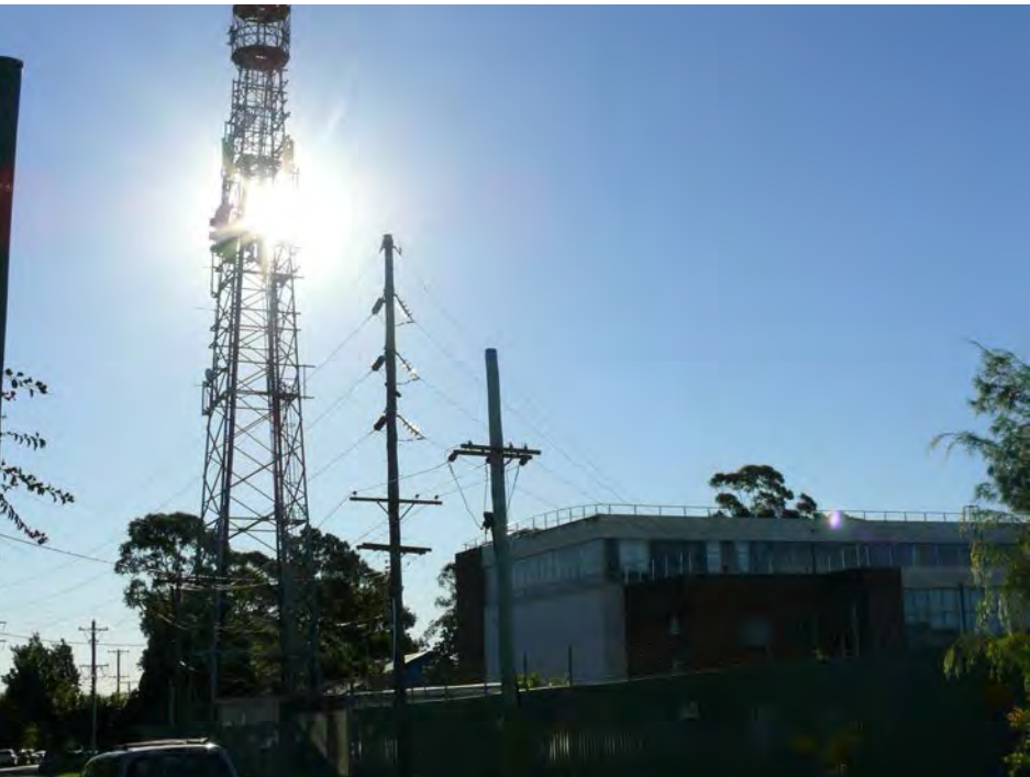
10 Looking to communications tower/substation
